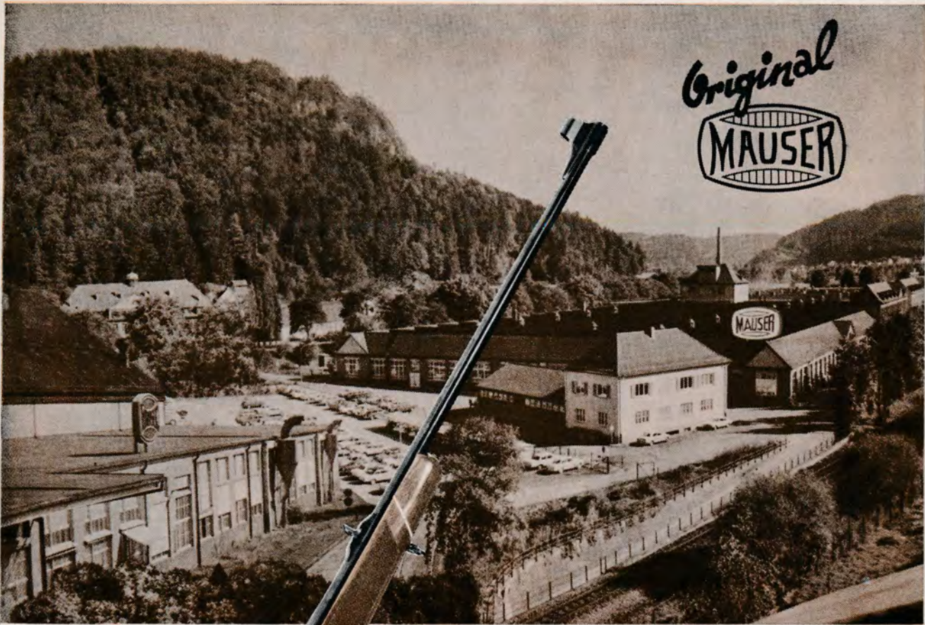
Partial view of the Mauser facilities in historic Oberndorf.
