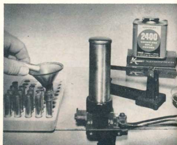
Experimentation showed 15 grains of 2400 to be adequate for the .444 shotshell loading.
