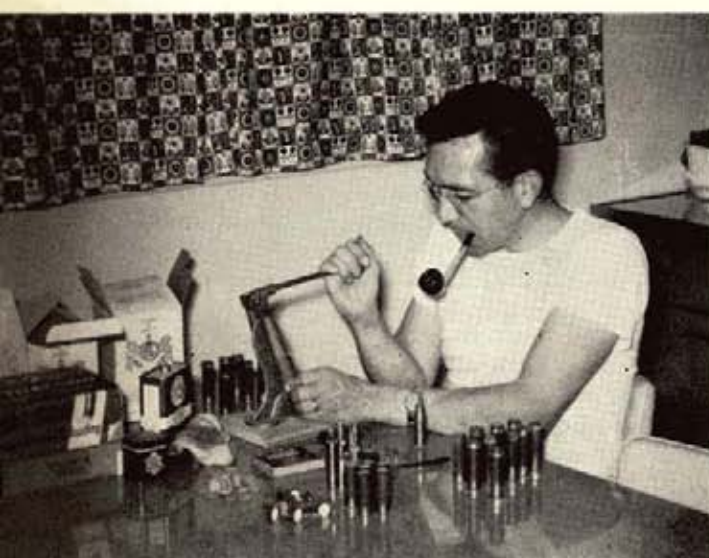
Neatly folded crimps finish off perfect reloads (left group), while batch at right are careless, scant on wad columns. Use of good tools like Thalsen (left) aids assembling accurate reloads.
