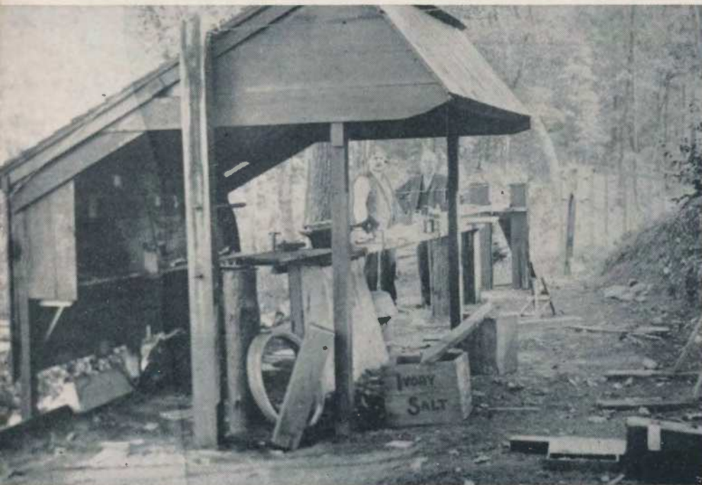
Dr. Mann's "Shooting Gibraltar." So named because of its heavy iron bed, laid in cement. On top of this was his test barrel on a "V" rest.
