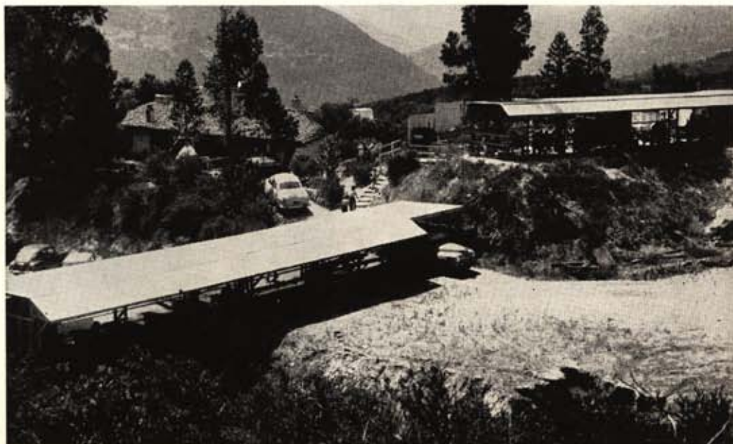
Firing points for big bore (right) and smallbore are roofed in cheap, cool aluminum to protect riflemen from the California sun.
