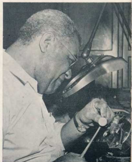
Left: Working on the cylinder of a Colt SA .45, Al Herbert is doing "plain engraving," which varies only slightly from gun to gun. Right: Deep lines require a hammer; shallow lines are cut manually.
