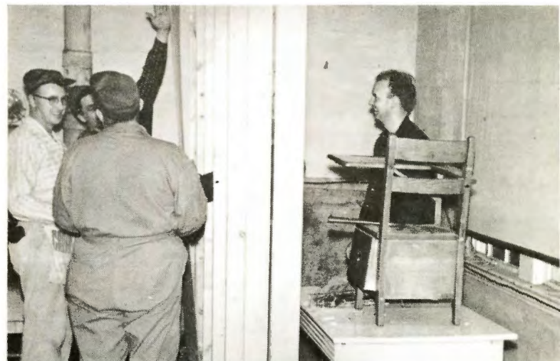
A work party of club members erected this separating partition between the club room and the firing line.
