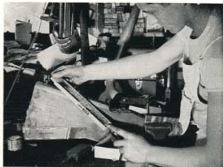
Surform black blade takes big chip, cuts fast for first hogging-out of stock from the rough blank, works like rasp.
