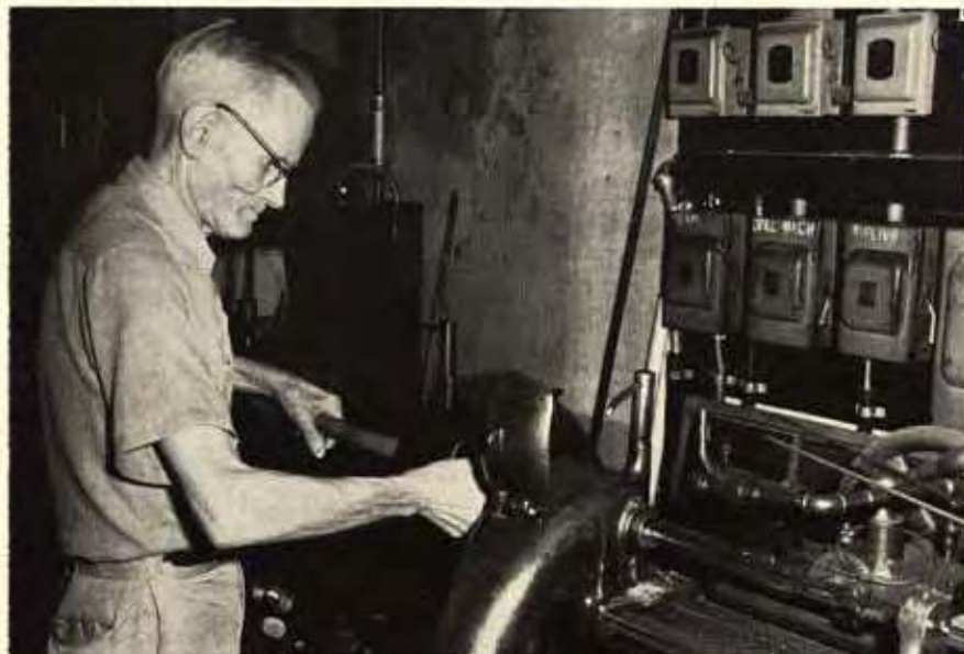
Master barrel-maker Eric Johnson, shown mounting barrel blank in deep-hole drill, is 71 years old, still active, still tough competition in any shooting match.
