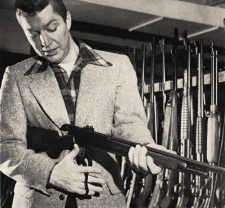
Watch lever rifles for wear on locking surfaces and correct headspace. Try a few shots to check extraction.
