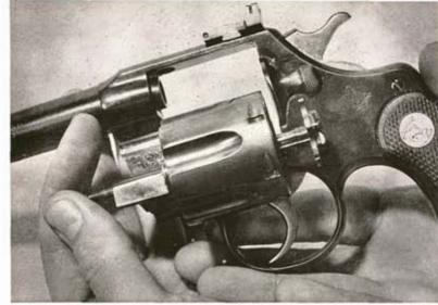
Side-swing loading used in 1866 Remington altered by W. C. Dodge is still used in modern-day Colt (right). Colt ratchet invented in 1836 (seen on end of rod) suffers battering on thumb latch, wears rapidly from careless closing.
