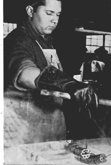
Finished cylinders are blued with nitrate bath after testing.
