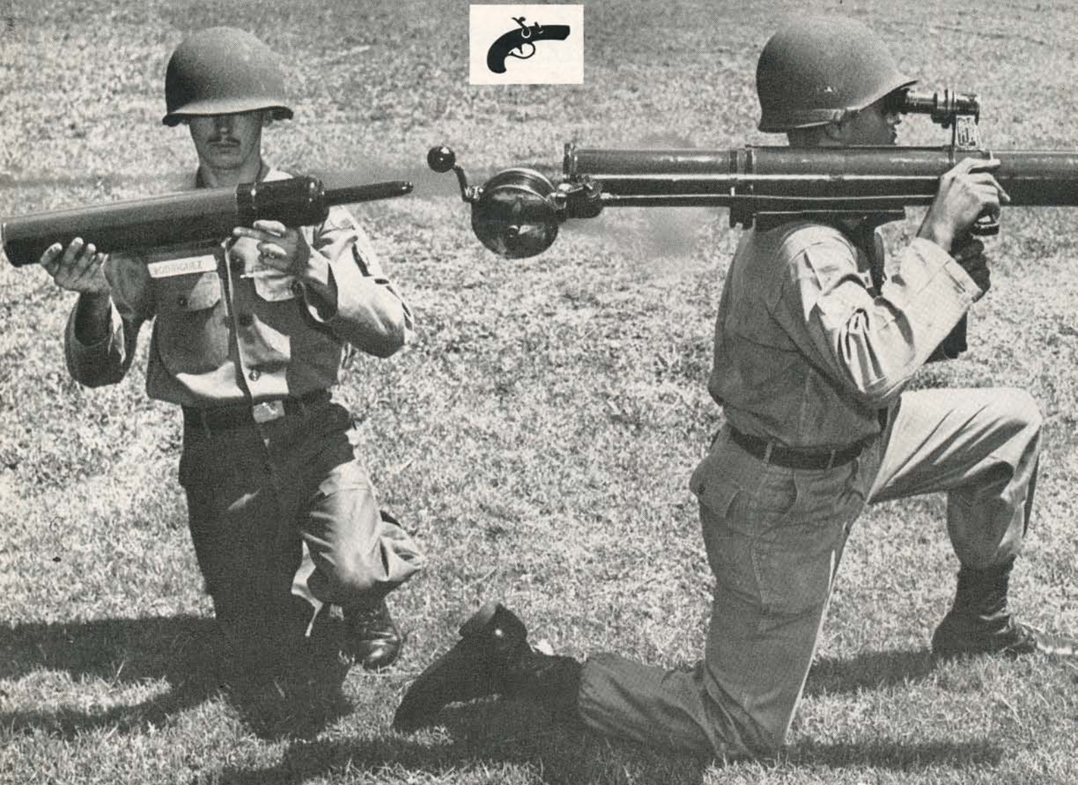
Recoilless rifle M 67, designed for use against tanks and armored vehicles weighs 35 lbs., can be fired from the shoulder, and requires only two men in field use.
