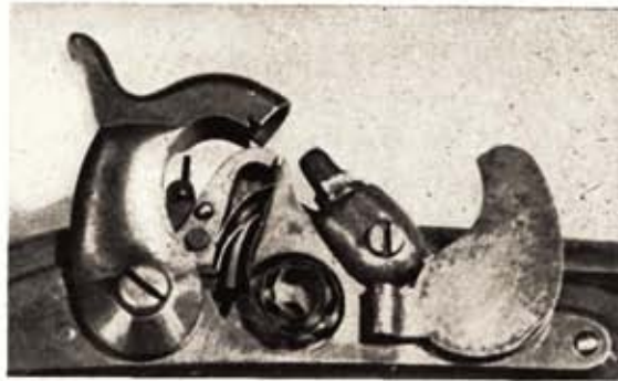
Richmond musketoon made by tools from Harpers Ferry Arsenal used unfinished salvage U.S. lock blanks forged for Maynard tape primer (right.)
