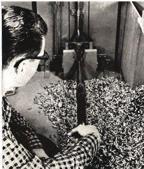
Factory test included 75,000 shots with no stops; plus 25,000 shots in dry gun.
