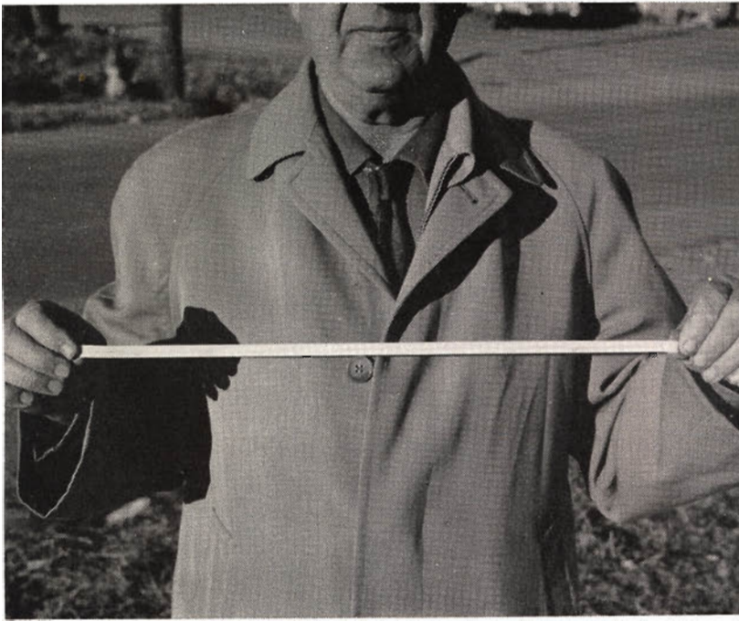
Loper holds paper timing tape with pen tracing which hits peaks when gun shot picked up by mike boosts current flow.
