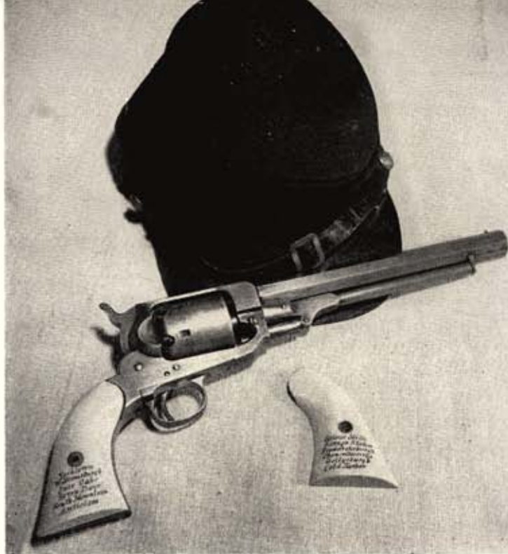
Mass-produced revolver made during Civil War by first Whitney Armory was all machine-made like today's guns.
