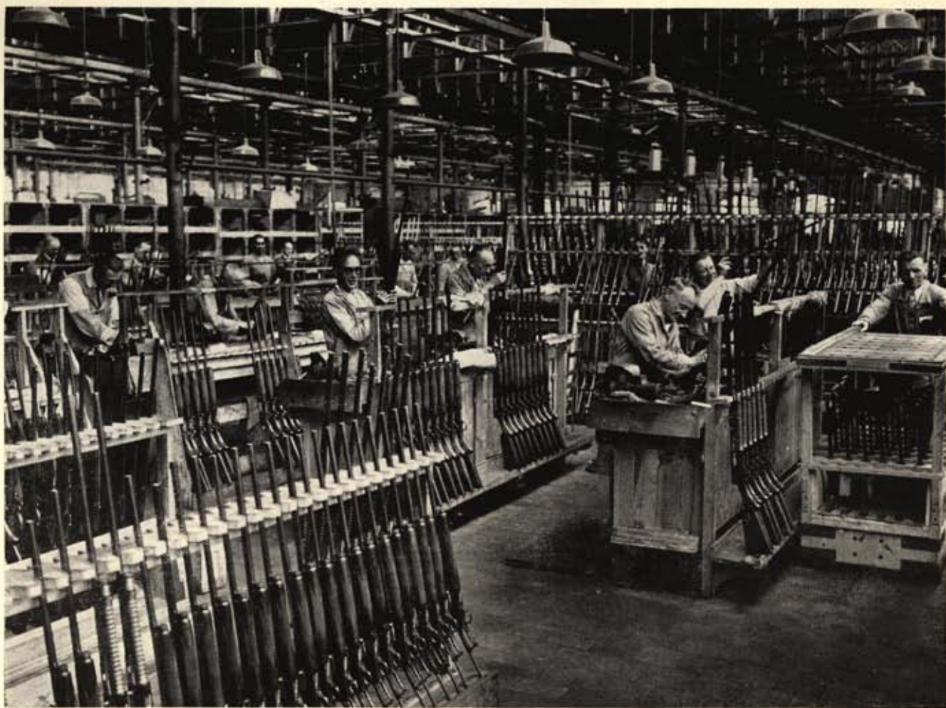
Huge factory in Belgium is where Browning guns are made. Overhead belts drive most machines. Hosts at Fabrique Nationale were director Laloux and young Browning.
