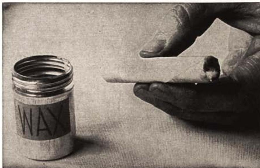
Tube was covered with outer wrap of stiff paper, powder poured in, and bullet inserted. Bullet end was crimped and dipped in hot lubricant of tallow and wax.
