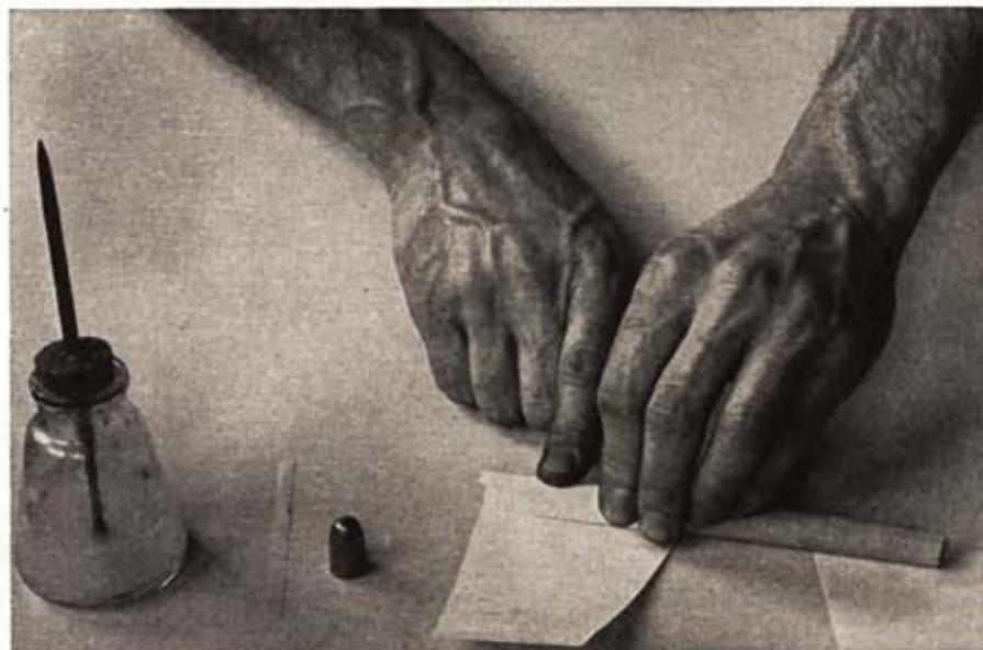
Two overlapping layers of thin paper were rolled over wooden mandrel to form tube. One end of tube was then folded over and fastened with paper strip.
