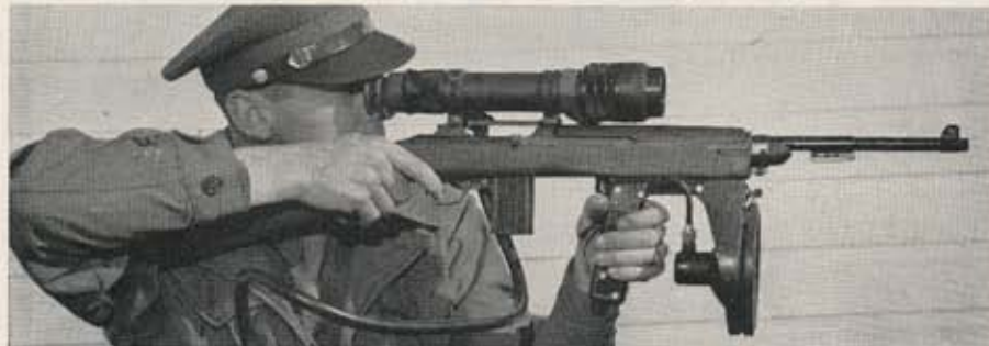
Snooper-scope has converter tube inside that changes invisible infra-red projected by stock flood light into image of target with phantom "V" sight in scope field.
