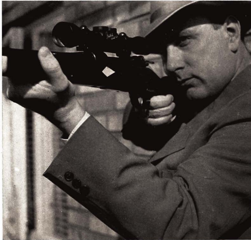
Kvale's converted 8 mm FN Mauser with Weatherby scope, firing 198 grain bullet at 2950 feet per second, is used by him for elk and other large game.
